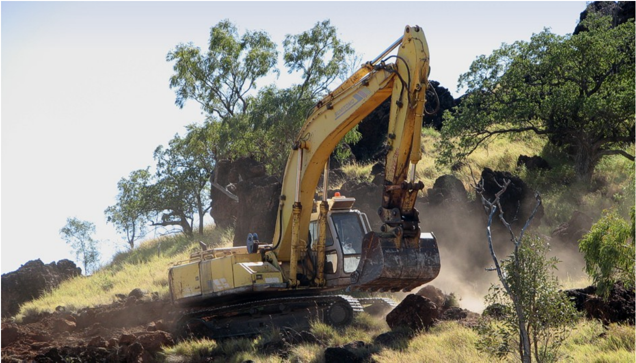
Fig 9: "Mozzie" clearing pads in difficult terrain at Wilgar. Limited access has hindered the exploration effort at Wilgar somewhat, with steep topography and rocky conditions severely limiting options for drill hole locations. A series of drill-pads are currently being cleared, to facilitate drilling from previously inaccessible locations.
